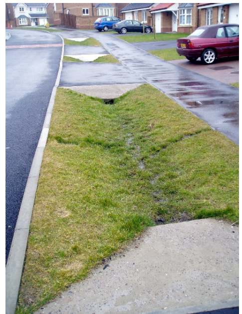
Figure 4-4. Photo of a swale. Credit: Susdrain .
