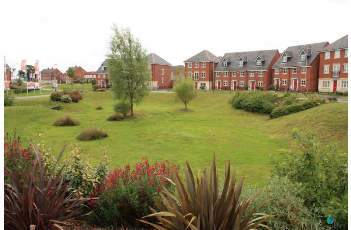
Figure 4-3. Photo of a detention basin. Credit: Susdrain .
