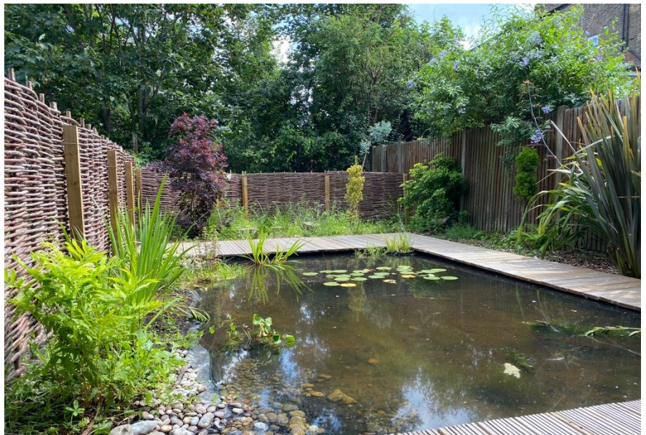
Figure 4-2. Photo of a SuDS pond. Credit: Meristem Design .
